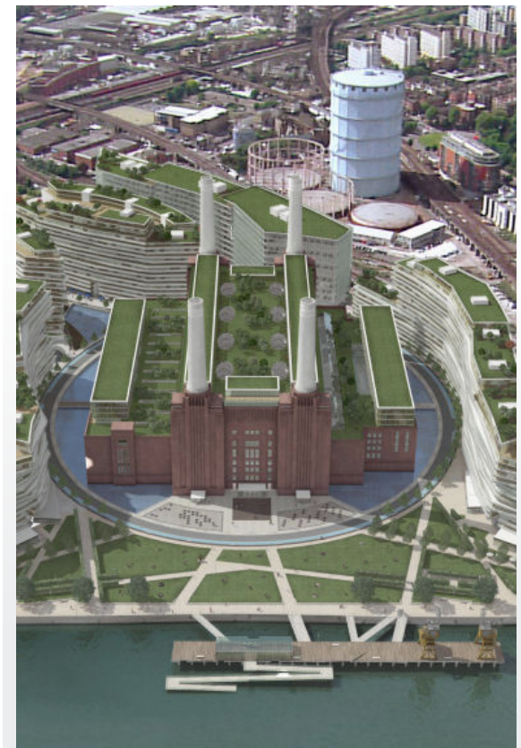
Figure 129 London's Battersea Power Station Green Roof
