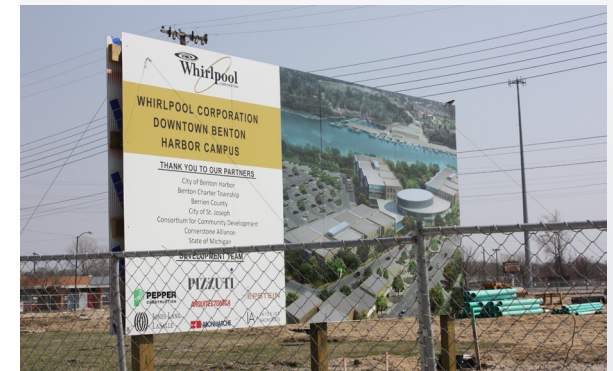
Figure 97 Benton Harbor Development
